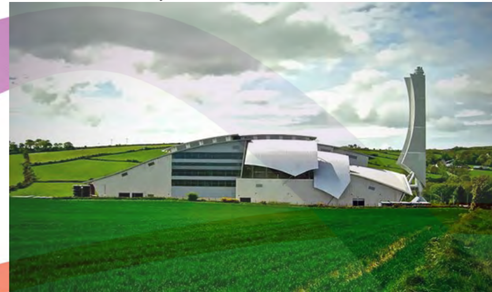
Isle of Man EfW facility
